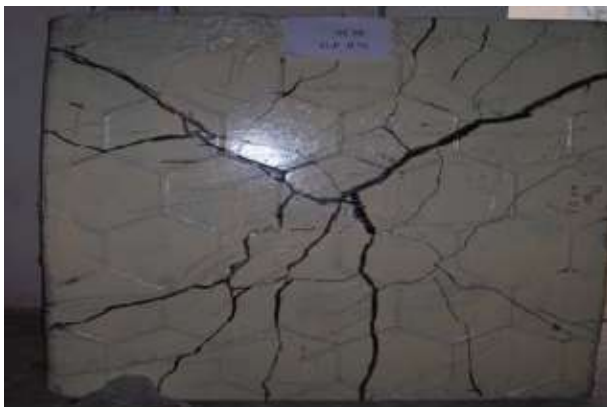
Slab 1 M 30 grade SCC with 0% glass fibres
