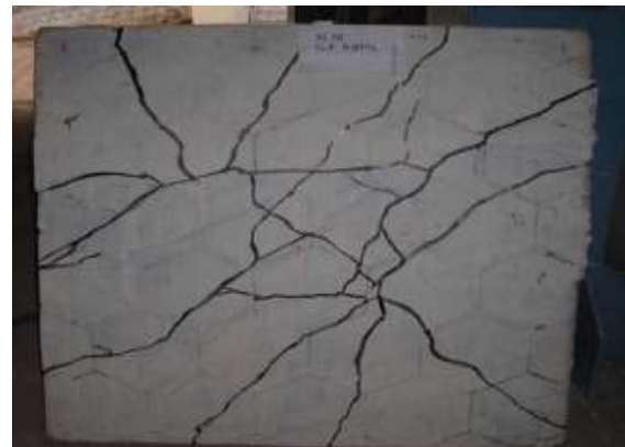
Slab 2. M30 grade SCC with 0.03% glass fibres
